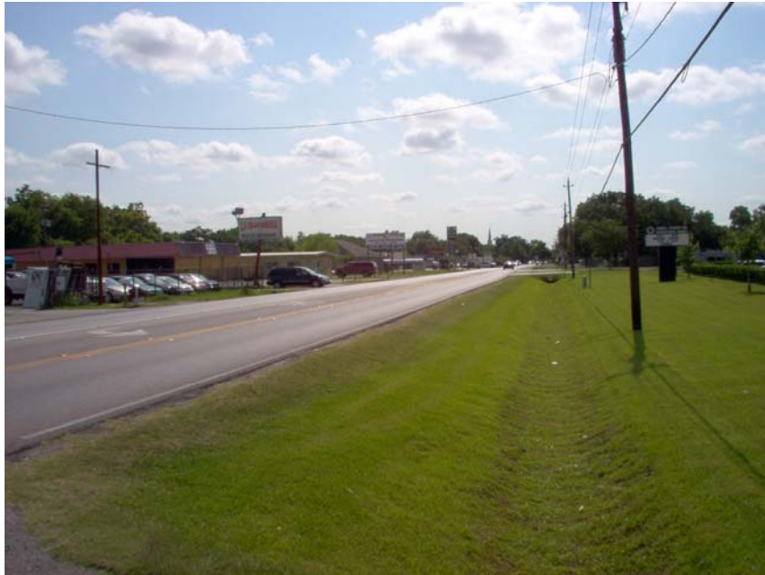
Picture 3.1: Ditch and Street Conditions on W. Gulf Bank Road
