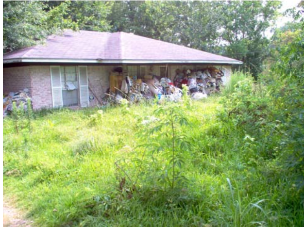
Picture 6.1: A Home in Violation of Public Health Codes
